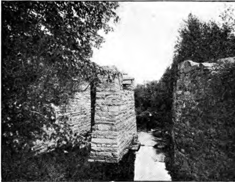
RUINS OF THE VIADUCT OVER SHAWSHEEN RIVER-- MIDDLESEX CANAL, 1755.
